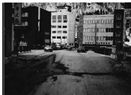
図31 月見橋の融雪状況 The snow melting appearance of Tsukimi bridge
